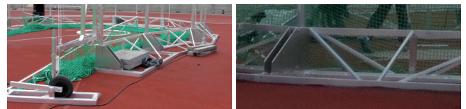
For a mobile safety cage: socket frame.
