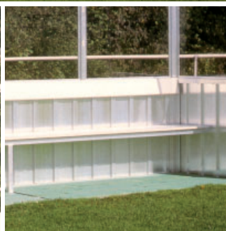
Seating area made of waterproof multiplex laminates.
