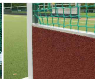
Moulded anti-noise coating
