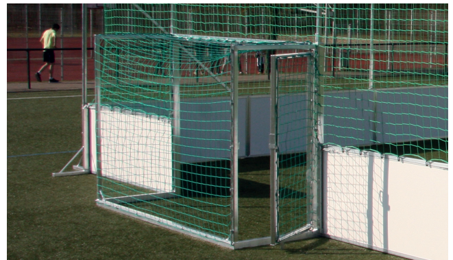
Corner reinforced with transversal strut.
